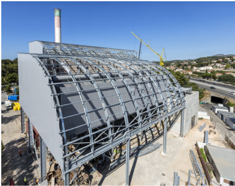
The curved roof of the Sittomat incineration and waste disposal plant takes shape.
