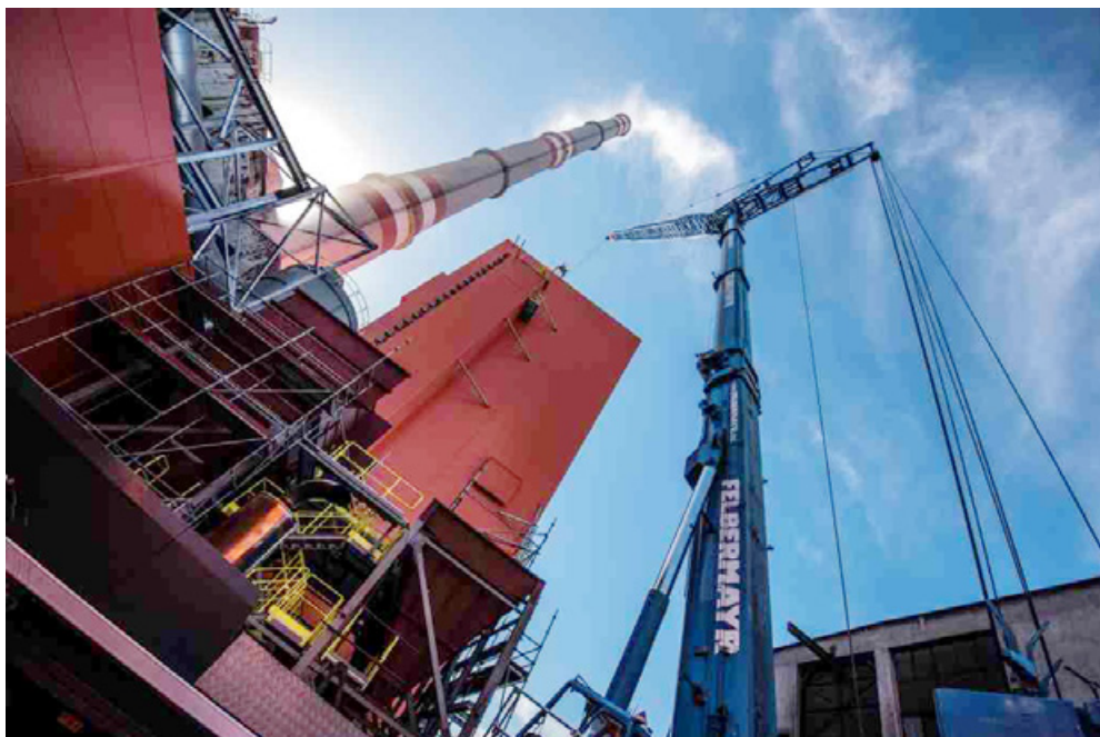
New fluid boiler being installed at ArcelorMittal Ostrava.
